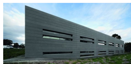
Figure 3.38 The narrow horizontal windows of the CEW Bean Building and concrete linear panel cladding. (Source: Denton Corker Marshall)
