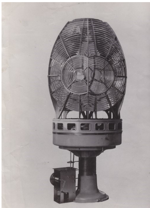
Figure 13. 1st Order Chance Bros. Lantern currently at Eddystone Point, ex. Cape du Couedic Lighthouse (Source: AMSA)
