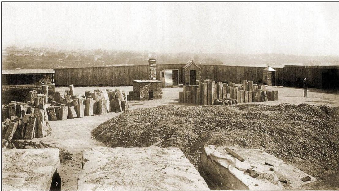
Figure 10: Sandstone quarried by the convicts was used to build many of the buildings on the island. It was also used for building works in Sydney, including the construction of Semi-Circular Quay. This photograph was taken in the 1890s during the second, or Biloela Gaol phase when prisoners who were capable of heavy work quarried and dressed stone in the paddock between the men's and women's sections.
